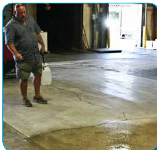
FIGURE 5-A: LAYING DOWN DENSIFIER WITH SPRAY TOOL.
