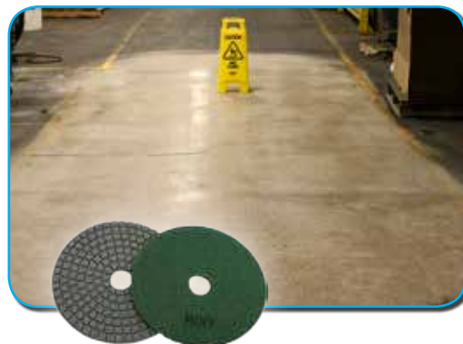
FIGURE 6-A: 800 GRIT GREEN SNAP! DISKS AND IMAGE OF FLOOR AFTER 800 GRIT DISKS.
