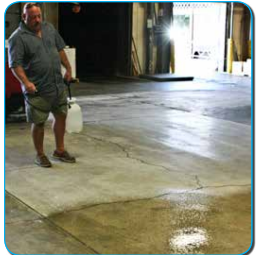
FIGURE 3-B: LAYING DOWN DENSIFIER WITH SPRAY TOOL.
