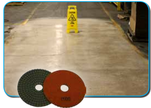
FIGURE 7-A: 1500 GRIT ORANGE SNAP! DISKS AND IMAGE OF FLOOR AFTER 1500 GRIT DISKS.
