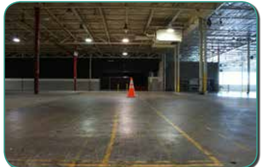
FIGURE 1-B: FLOOR STARTING POINT. NOTICE THE NONUNIFORMITY AND SCRATCHES/GOUGES.
