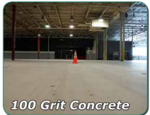
FIGURE 1-E: AFTER 100 GRIT CONCRETE PREP TOOL.
