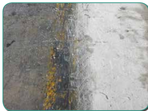
FIGURE 2-A: UNIFORM WHITENING ON THE CONCRETE WILL BE VERY NOTICEABLE. IF NOT - CONTINUE PROCESS TILL FLOOR IS UNIFORM.
