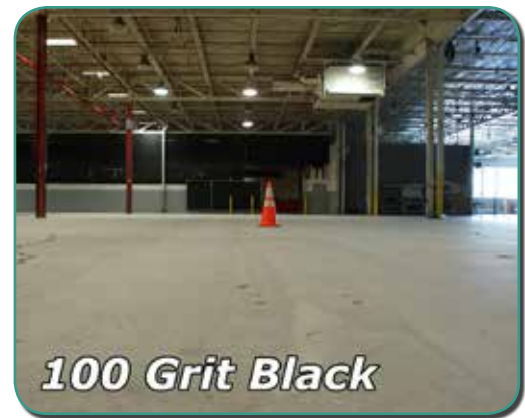
FIGURE 3-A: EITHER STARTING AT THIS POINT TO ESTABLISH A BASE POLISH OF THE FLOOR OR THE FLOOR HAS JUST ADVANCED FROM LEVEL 1.
