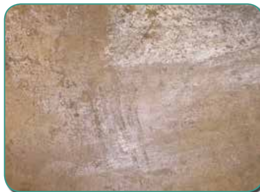
FIGURE 4-B: LEAVING DENSIFIER ON THE FLOOR TOO LONG CAN CAUSE DISCOLORIZATION.
