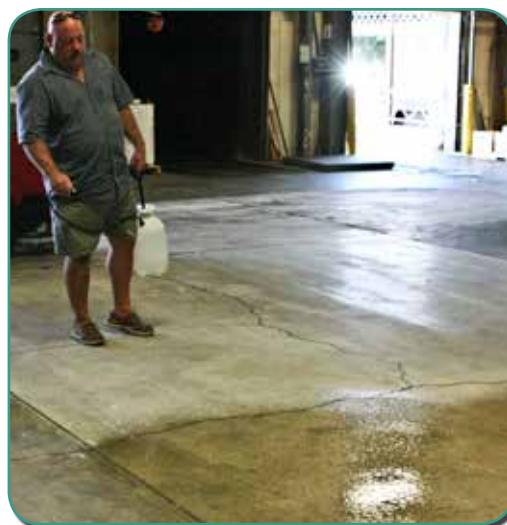
FIGURE 4-A: LAYING DOWN DENSIFIER WITH SPRAY TOOL.
